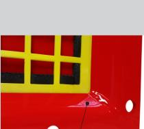
45° degree flange on interior of door prevents fines from accumulating.
