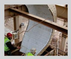
ASGCO® X-WEAR™ is a resilient wear resistant panel made up of High Density Abrasion resistant Ceramic bonded to a mild steel backing plate with impact resistant urethane compound. It easily out performs steel, chromium carbide overlays and conventional ceramics.
