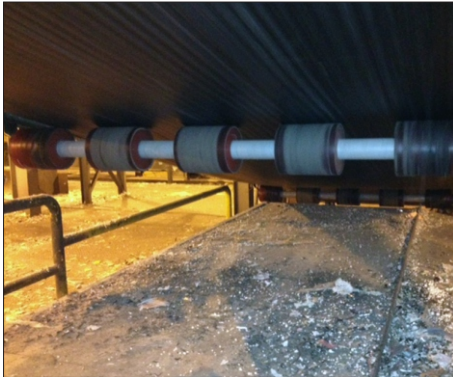
Dura-Sleeve™ Idler Installed
