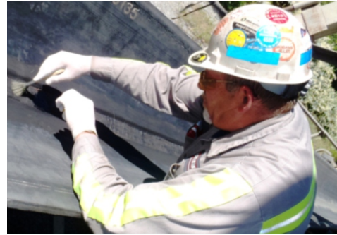
Applying cleaner and primer.
