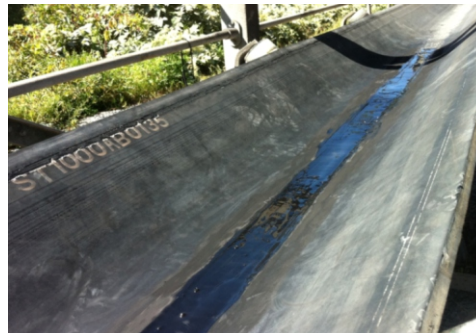
Finished. Longitudinal groove repaired.
