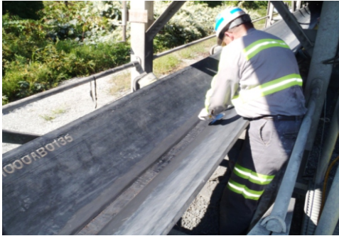
Grinding/Cleaning old rubber out of damaged conveyor belt.
