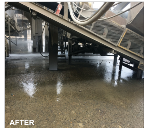
AFTER Clean floor after installation of Mini-Skalper ® IV.
