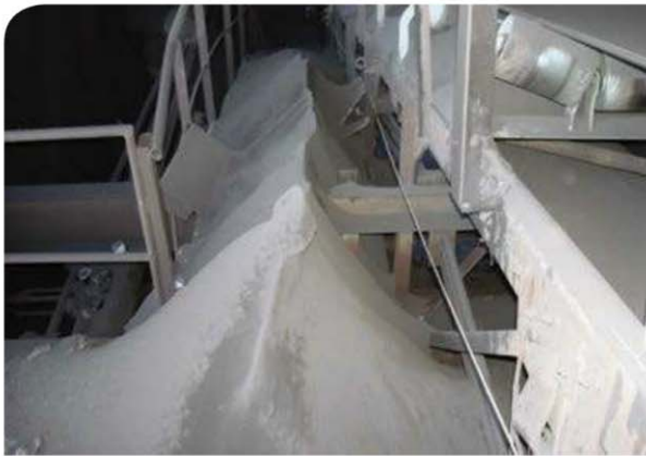
Figure 1. Material spillage at the load zone.
