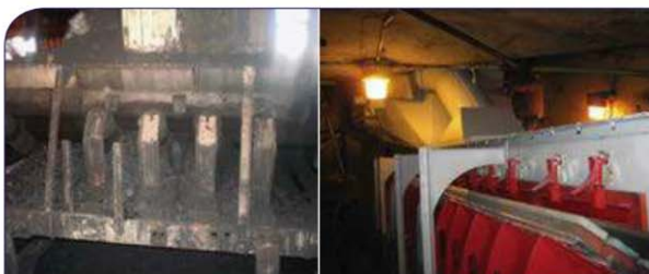
Figure 3. Before and after pictures of a complete Transfer Point rebuild.
