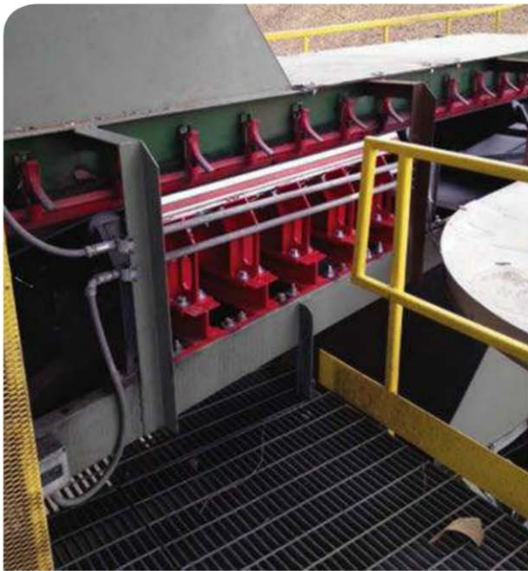
Figure 5. Example of proper belt support, wear liners and skirting.
