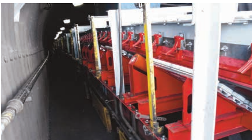
Figure 3. Secondary load point and full length skirt tunnel.
