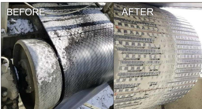
Lower Bend: Before and After
