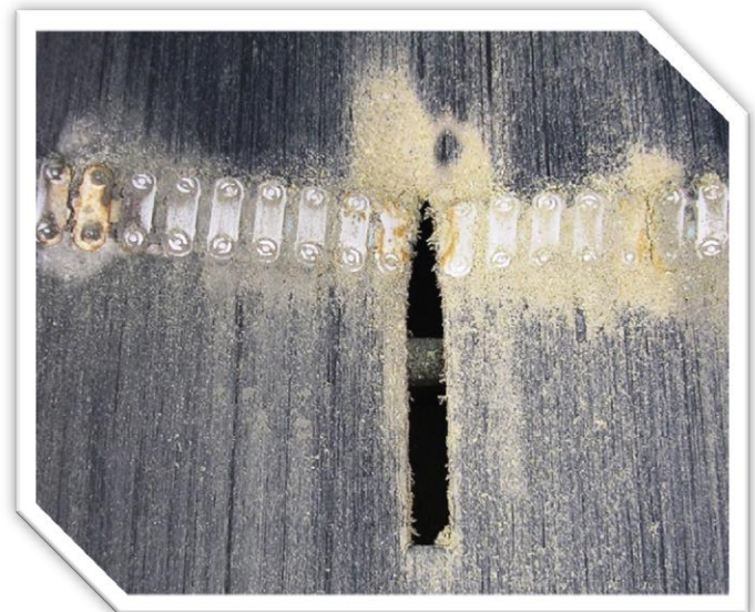
Pictured is a failing mechanical splice.
