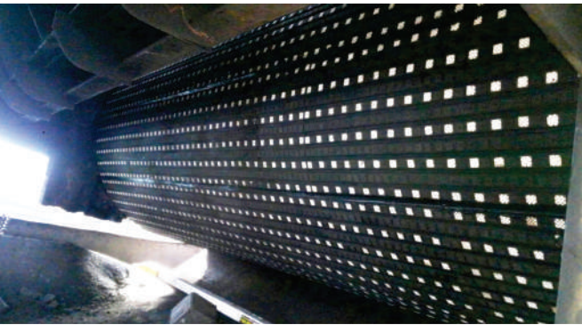
Arrowhead Rubber Pulley Lagging - Bulk Shipping Terminal Installation
