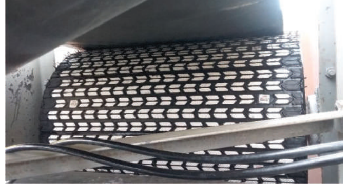
Arrowhead Ceramic Pulley Lagging - Asphalt Plant Installation
