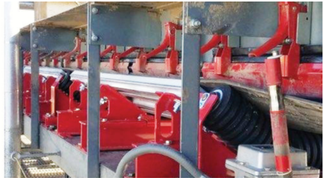
AFTER WITH ASGCO COMPONENTS.
