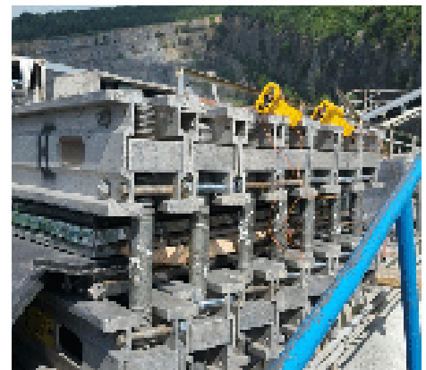
ASGCO ® 's Vul-Con ® vulcanizing press is set-up on the conveyor to cure the belt.
